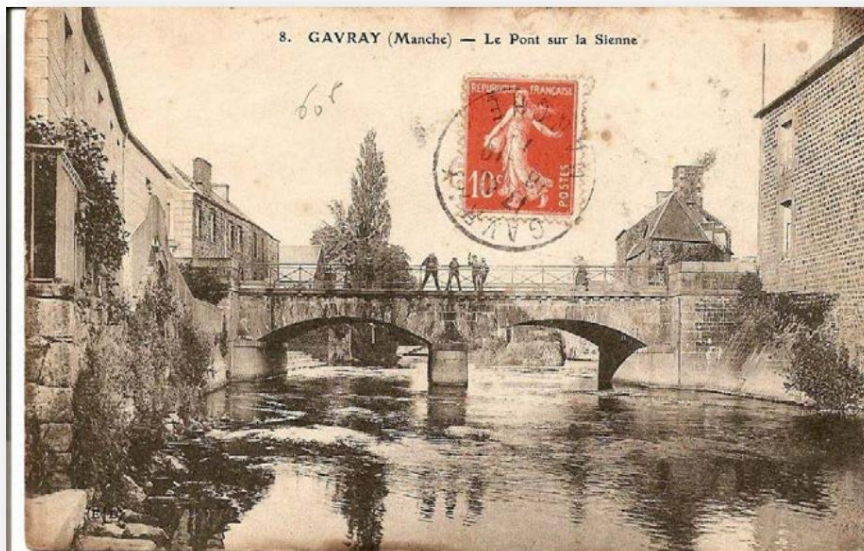
22 The bridge over the Sienne
